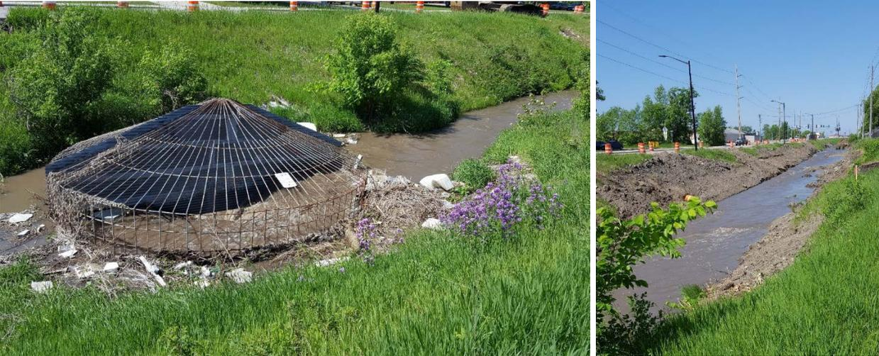
During June runoff, a plume of sediment was found to be entering the Thief River upstream of the Hillyer Bridge (140<sup>th</sup> Ave NE). A fresh bank failure and streambank erosion also developed downstream of the bridge.
